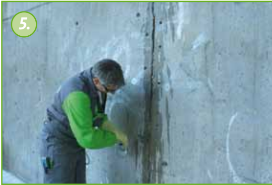
Pre-wet the crack
