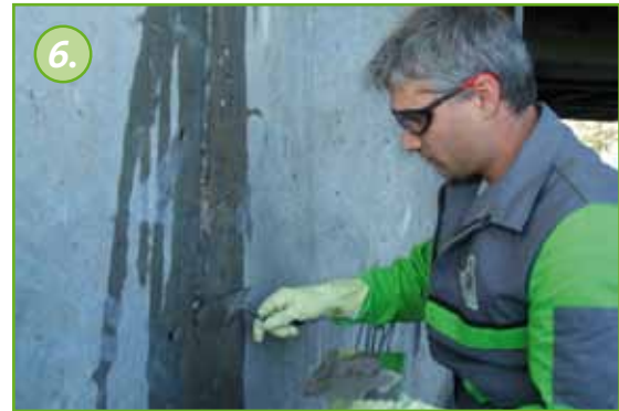
Close the crack along its course with KÖSTER KB Fix 5. Closing the crack prevents injection material from prematurely flowing out of the crack during the injection. Setting time is approx. 5 minutes, depending on the surrounding temperature and humidity.
