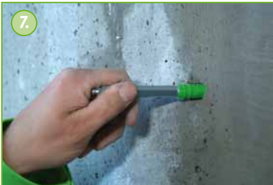
Install KÖSTER Superpackers in the boreholes leaving about every third borehole open.
