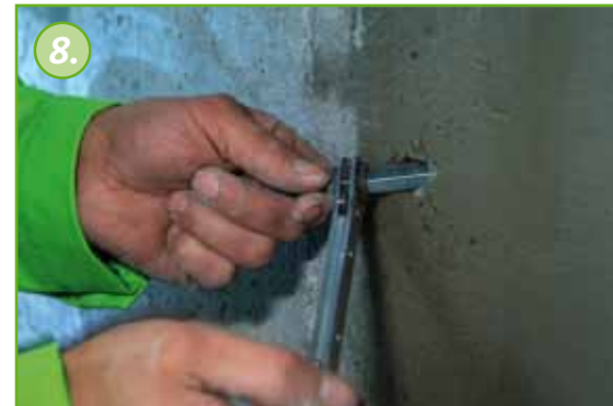
Use a wrench to tighten the packer.
